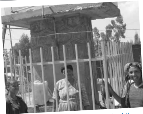
5. Part of the WaterCan project involved the construction of a reservoir on top of this distribution point, allowing water to fill up at night, providing access all day long.
