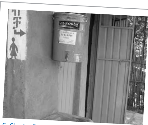
6. Chesire Foundation constructed hand washing facilities as part of the latrine.
