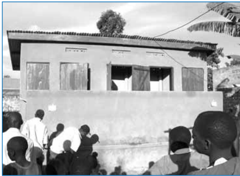
A community "ecosan" toilet block nears completion.
