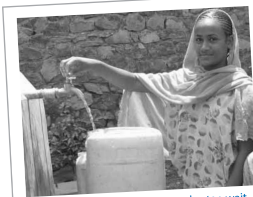
1. Constructed with four taps to shorten wait times, the standpipes allow containers to be rested during filling, and runoff to be directed to vegetable gardens and cattle troughs.
