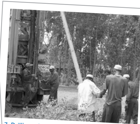
7. Drilling a borehole well.
