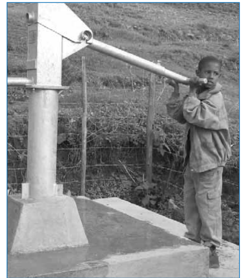
Deep well hand-pump models such as this rugged Afridev, and the India Mark II and U3, are conventional lever action models, and are commonly found in WaterCan projects.
