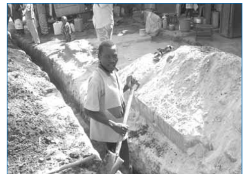
Residents help dig trenches for water feeder pipes.
