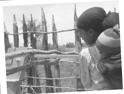
8. A pump with a twist - two branches laid horizontally act to restrict the range of motion of the pump and extend its lifespan.
